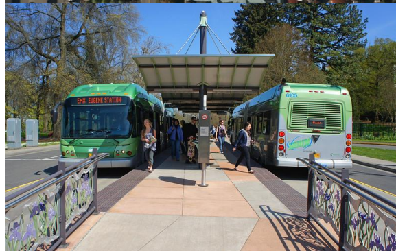
Double track center running dedicated EmX lanes in Eugene to alleviate existing capacity challenges
