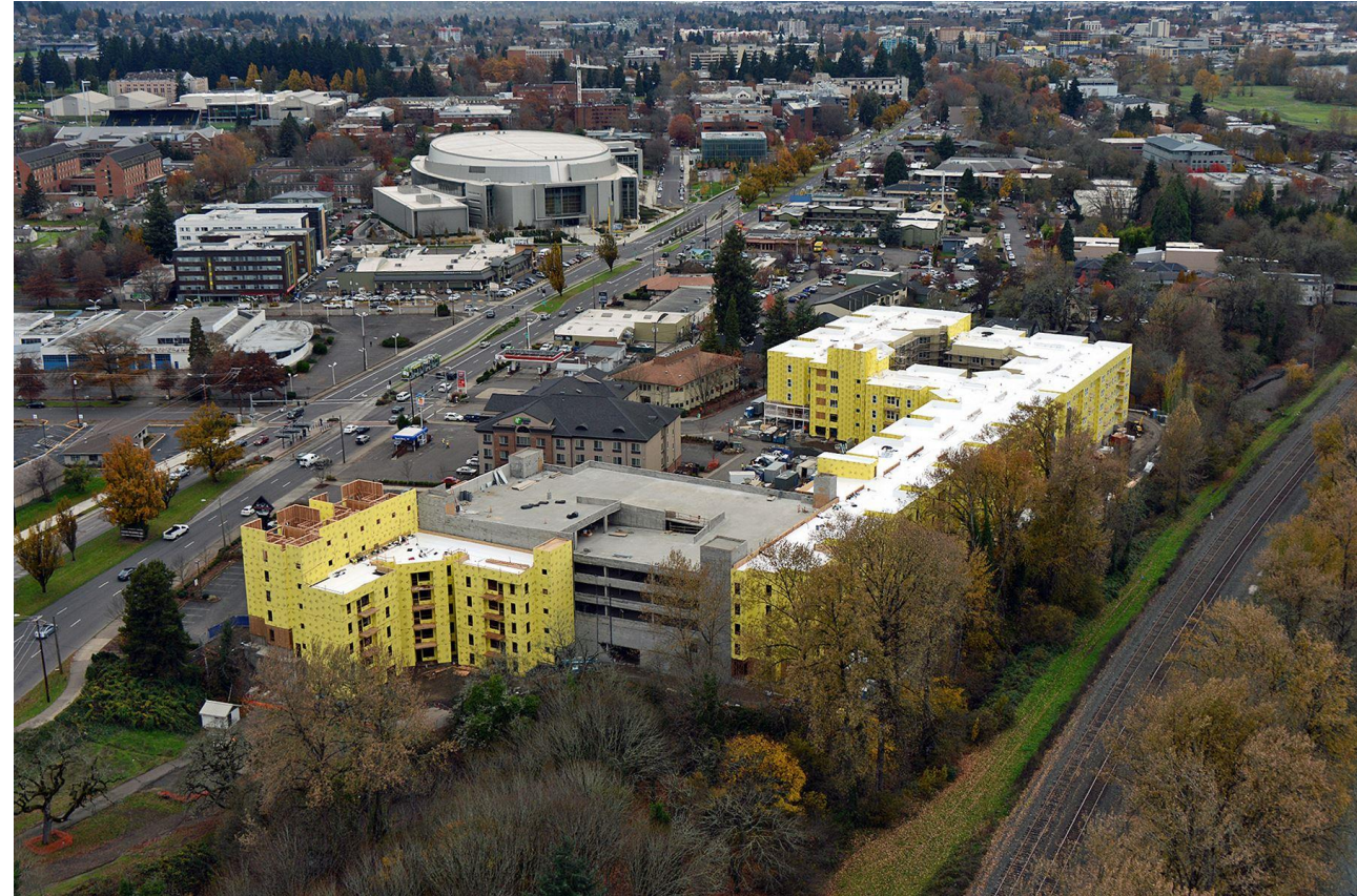
Drone Construction Photo
