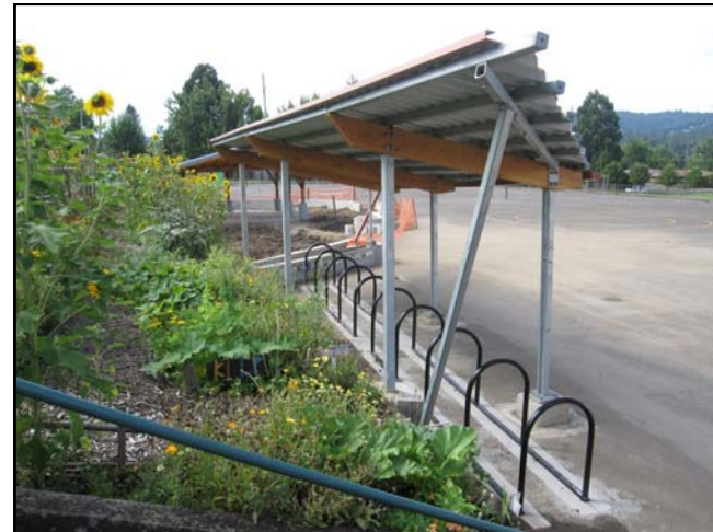
Camas Ridge Covered Bicycle Parking with Rainwater Catchment System. Photo by Shane MacRhodes.
