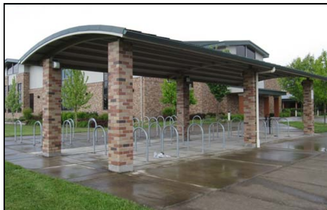
Covered Bicycle Parking at Madison Middle School. Photo by Shane MacRhodes
