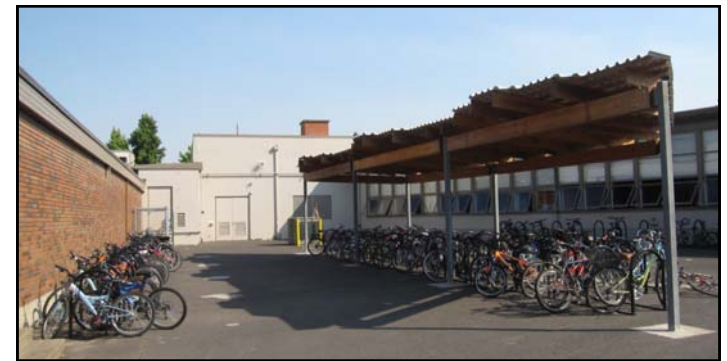
Upgraded Covered Bicycle Parking at Roosevelt Middle School. Collaboration Project with University of Oregon
