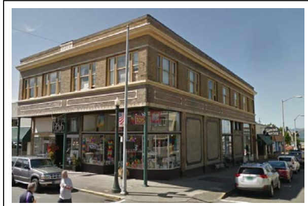
Figure 14.158-4: Base, Middle & Top of Building
