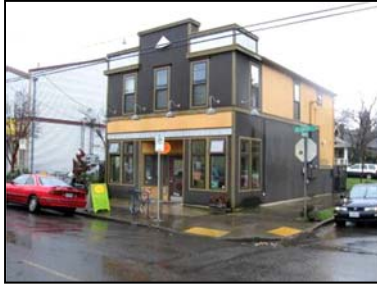
Figure 32 Top of building features a parapet
