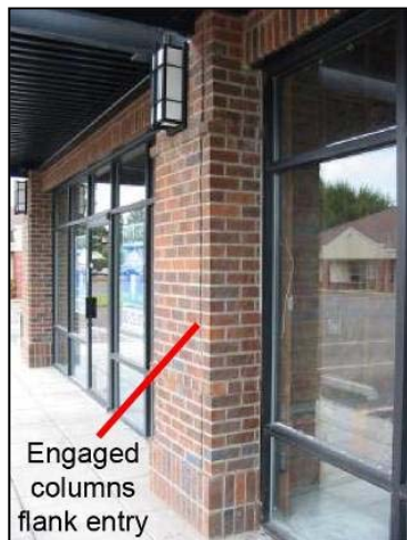
Figure 43 Entry flanked by engaged columns and lighting
