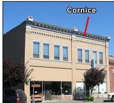
Figure 58 Cornice used on flat roof
