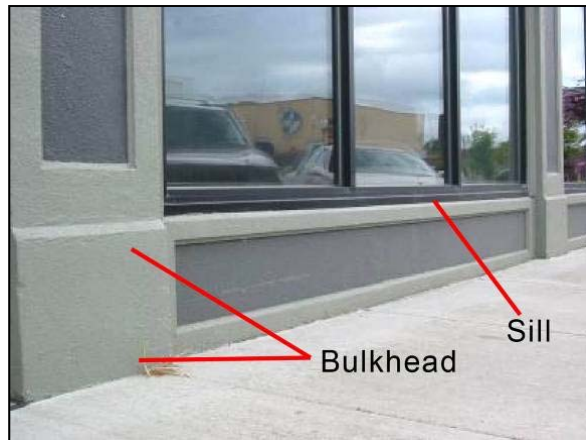
Figure 54 Building base elements
