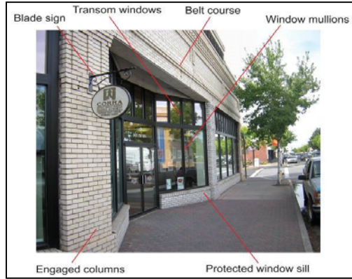
Figure 49 Design elements for bays
