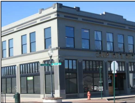
Figure 19 Design details such as a recessed entry, columns and decorative transom windows help articulate the ground floor and distinguish it from the upper floors
