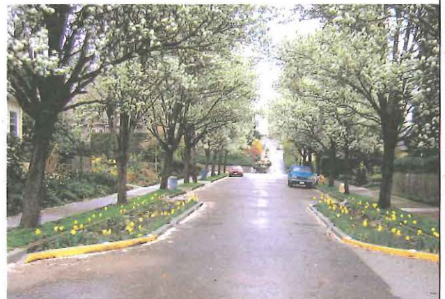
Stormwater Curb Extension (NE Siskiyou St, Portland)
