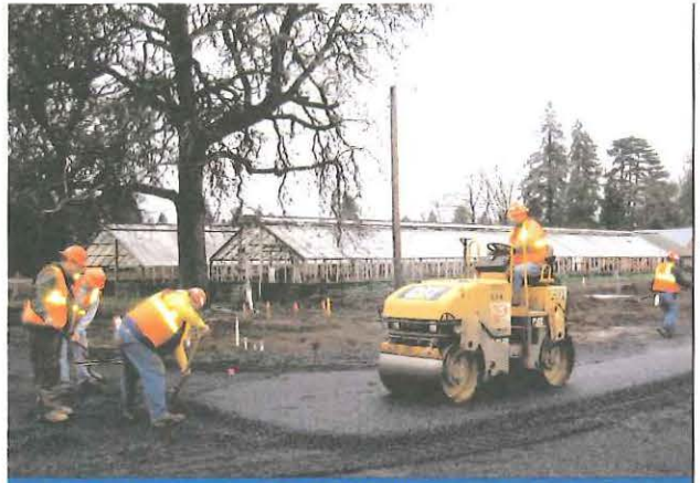
Pervious Pavement (Pringle Creek Community, Salem)
