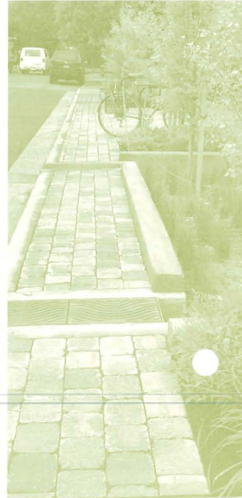
Stormwater planters collect and treat stormwater on site, allowing runoff to soak into the ground.
