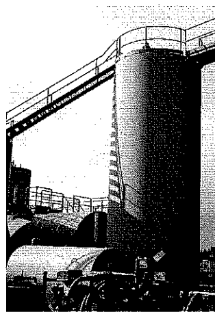
Local clean-diesel storage tanks make project a success.
