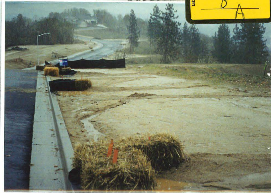
Photograph Four Turbid water flowing past barrier
