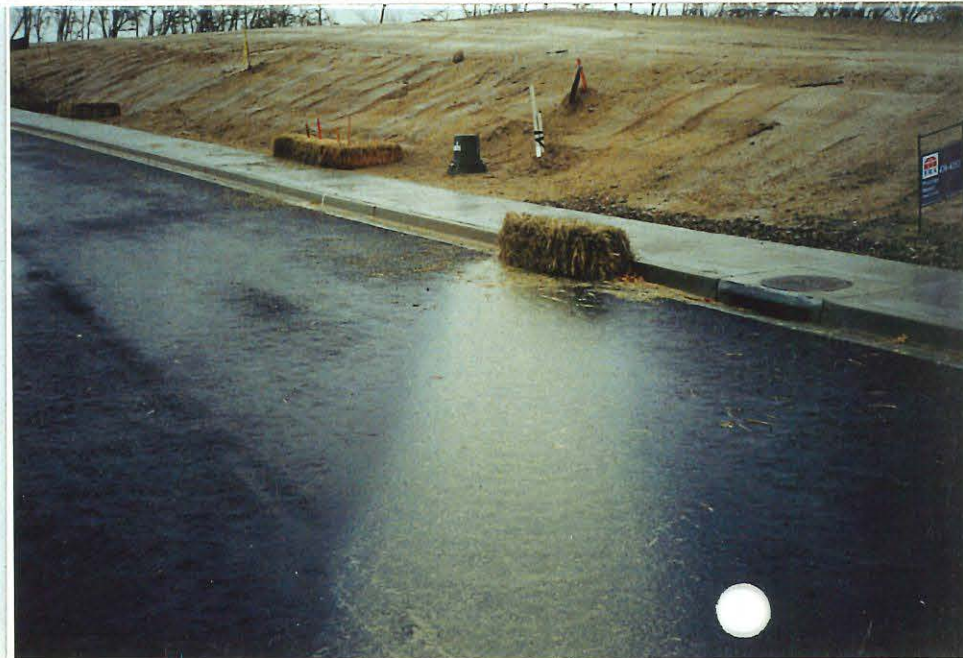
Photograph Twelve Turbid water flowing past barrier
