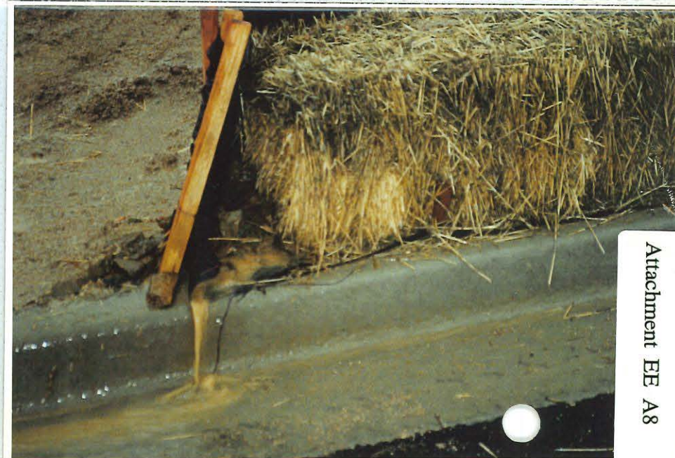
Photograph Four Turbid water flowing past barrier
