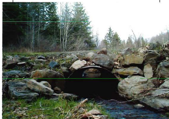
A pipe-arch culvert used on a tributary of Clear Creek eight miles south of Estacada is one example of responsible riparian management under the Oregon Plan for Salmon and Watersheds. The landowner is Port Blakely Tree Farm.
