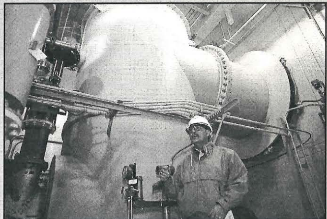
Nerve and blister agents will be destroyed in the liquid incinerator.
