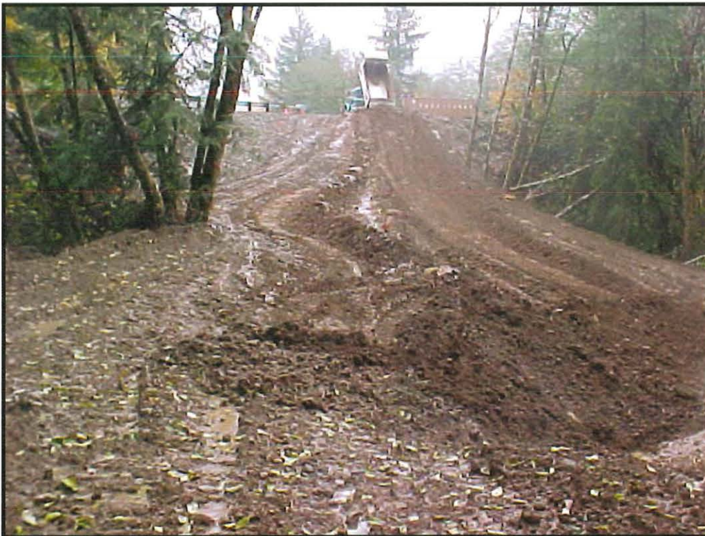
Treated soil being used to fill and regrade the spill site.
