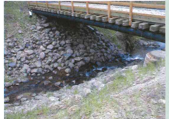
Boxler Creek now provides fish passage after installation of a bridge.
