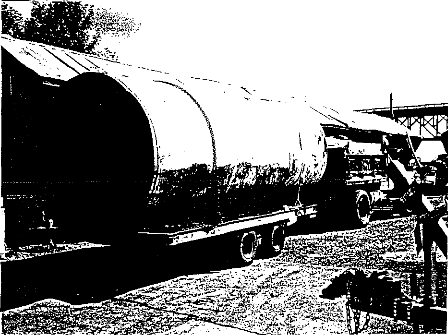
Transporting USTs to recycling facility. USTs have been labeled and rendered unusable.
