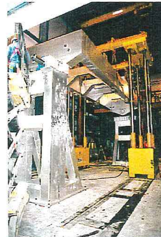
75% Mechanically Complete Test and Checkout Underway
