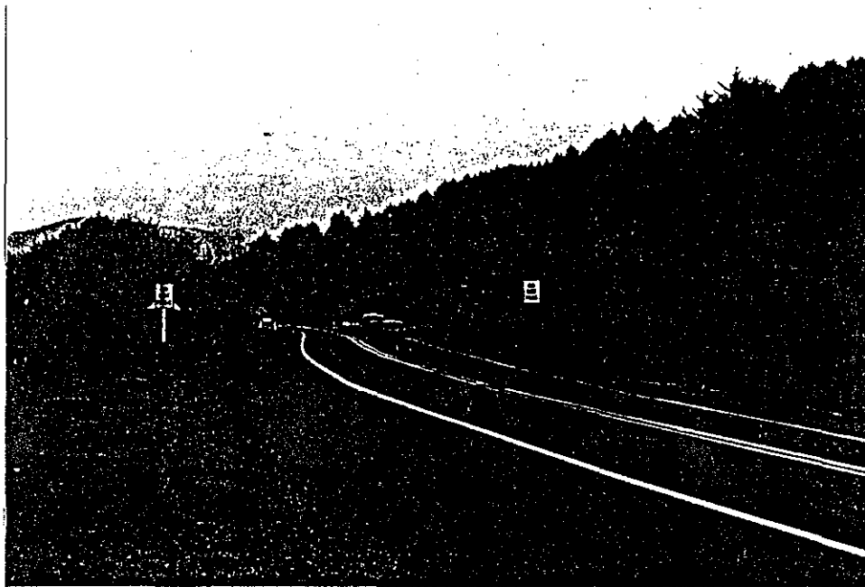
Photo #7 View north along highway. Shear coincident with beginning of fresh paving. Automobiles at approximate crest of bulge.
