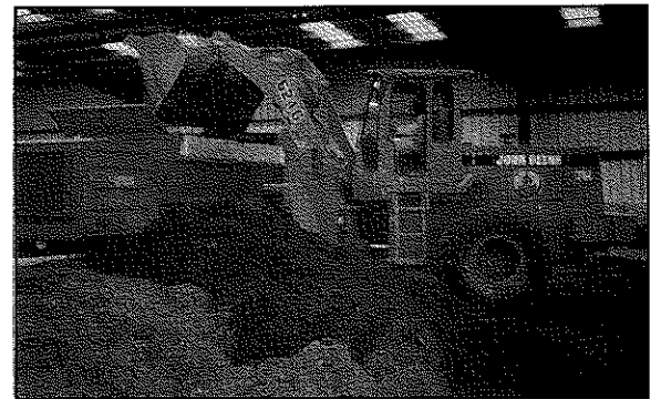
Soil and ingredients are moved inside the treatment building where the process begins.
