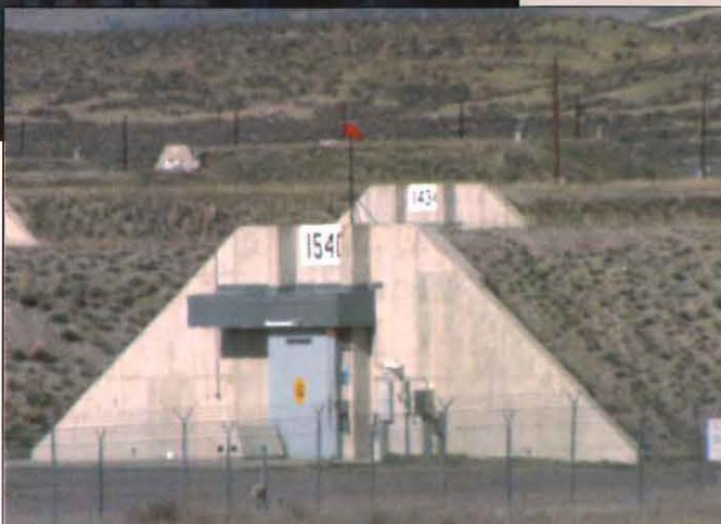
Earth-covered igloos provide secure storage of weapons near the facility.
