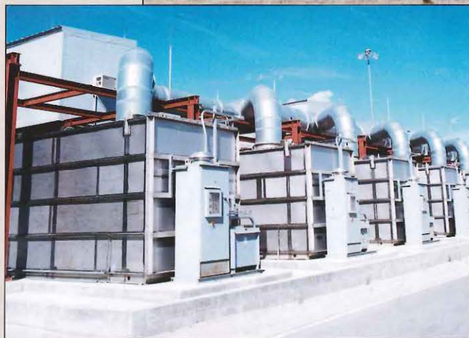
Multiple carbon filters provide an added layer of protection by cleaning plant air before it is released to the environment.
