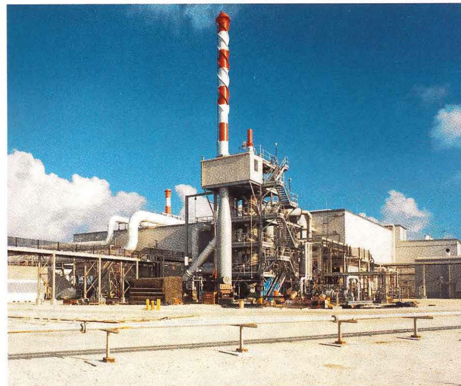
Discharges from the stack are continuously monitored and must meet the requirements of the Clean Air Act.
