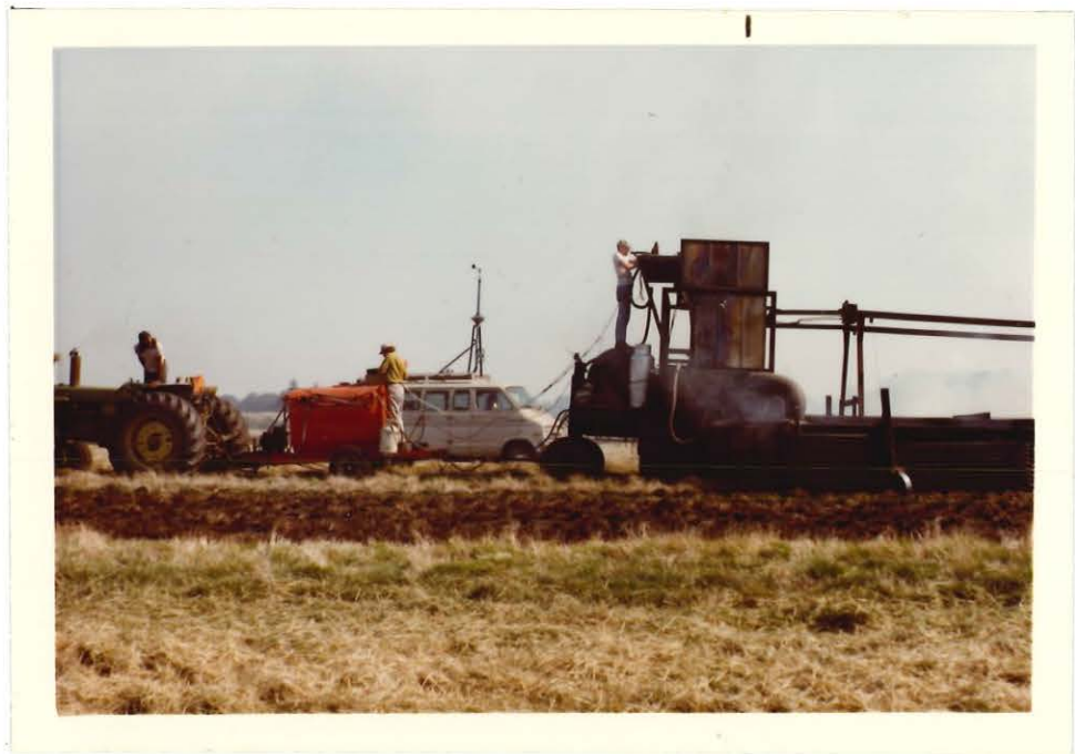
Testing stack and fugitive emissions on Sanitizer #75-02 operating in a heavy stubble perennial ryegrass field in 1976.
