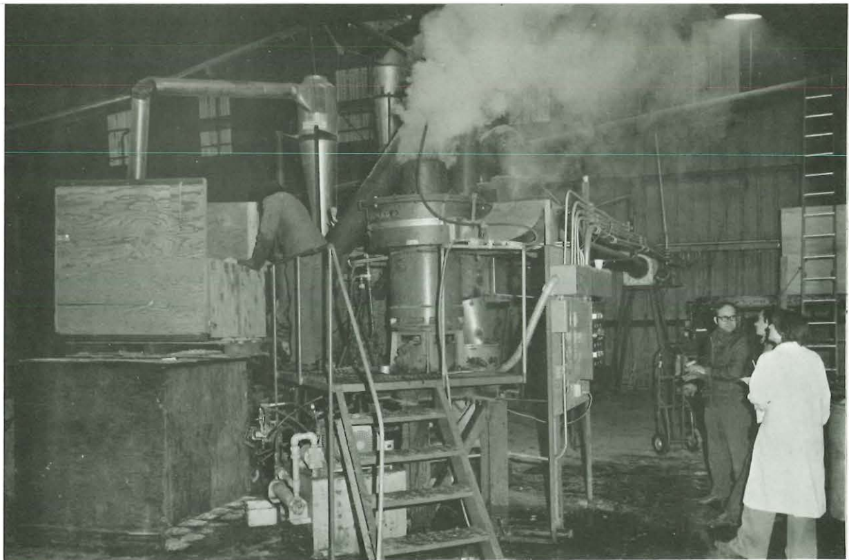
Presteamed straw being defiberized in the Committee's disc refiner pilot plant at Straw Center. Contiguous straw-fired fiber drying loop in background uses same straw as fuel.
