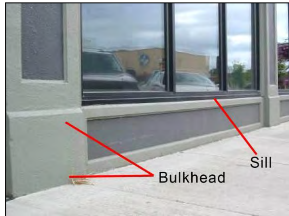
Figure 54 Building base elements
