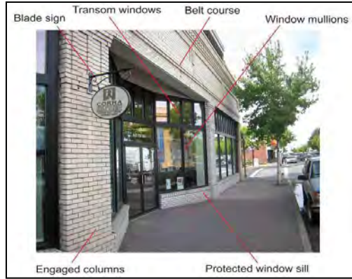
Figure 49 Design elements for bays
