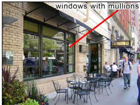
Figure 53 Elements of the bottom of the building
