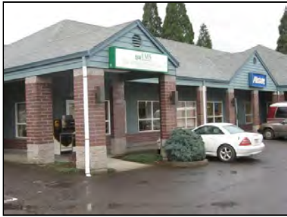
Figure 27 Examples of development in the Outer Highway Commercial sub-area
