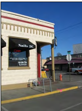
Figure 31 Cornice details near the top of building
