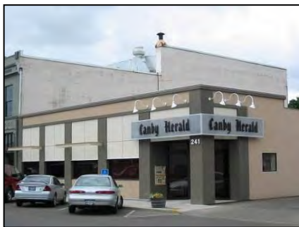
Figure 24 The Canby Herald Building in the commercial core incorporates many good design elements including a recessed entry, sign frieze, engaged columns and decorative lighting
