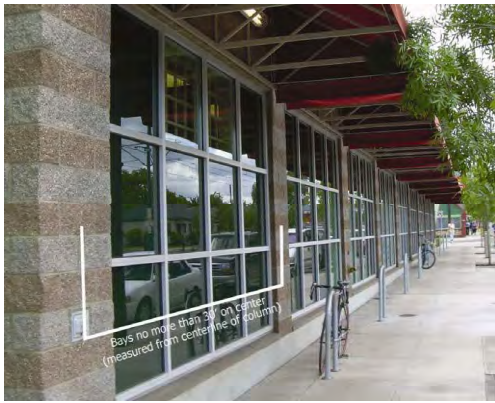
Figure 29 Repeating bays with a continuous awning
