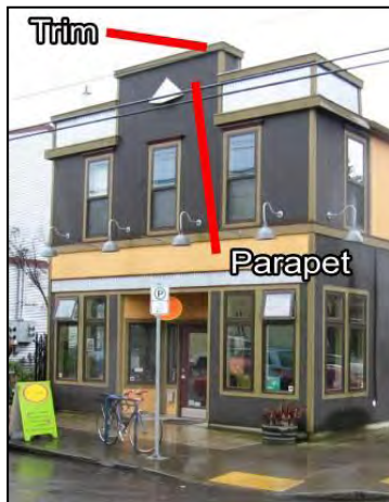
Figure 59 Parapet used on flat roof
