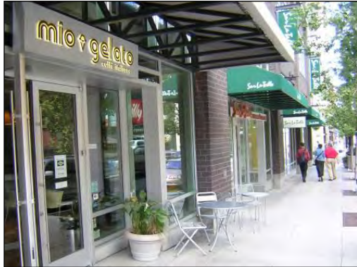
Figure 3 A high degree of transparency (windows) helps create a sense of interaction between activities inside and outside the building
