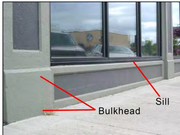
Figure 54 Building base elements
