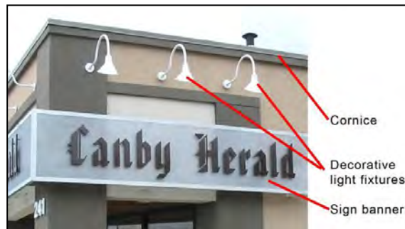
Figure 55 Middle and top of ground floor elements
