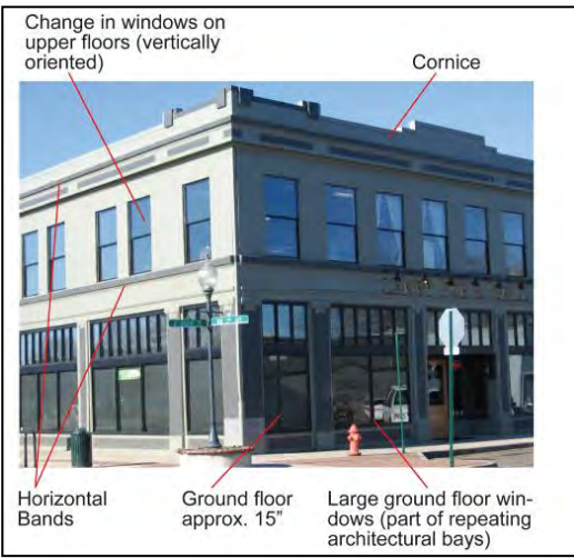
Figure 51 Example of distinct bottom, middle & top of building
