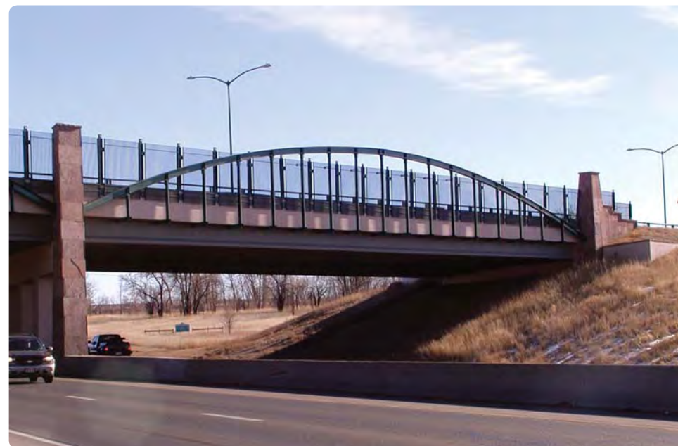
Architectural iron work added to picket style fencing
