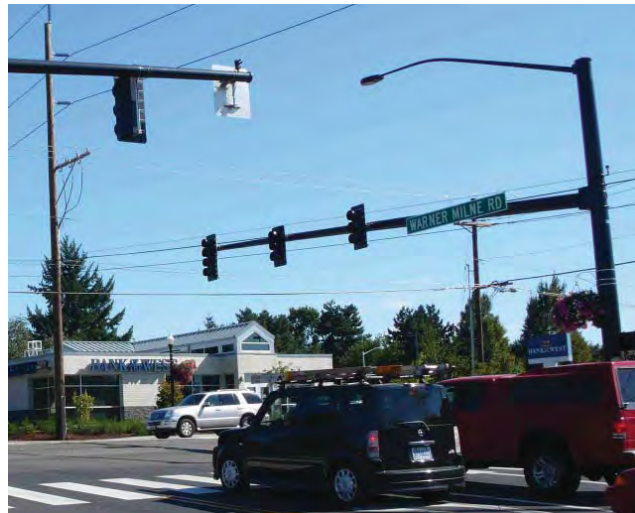
ORNAMENTAL SIGNAL POLES AND MAST ARM EXAMPLE
