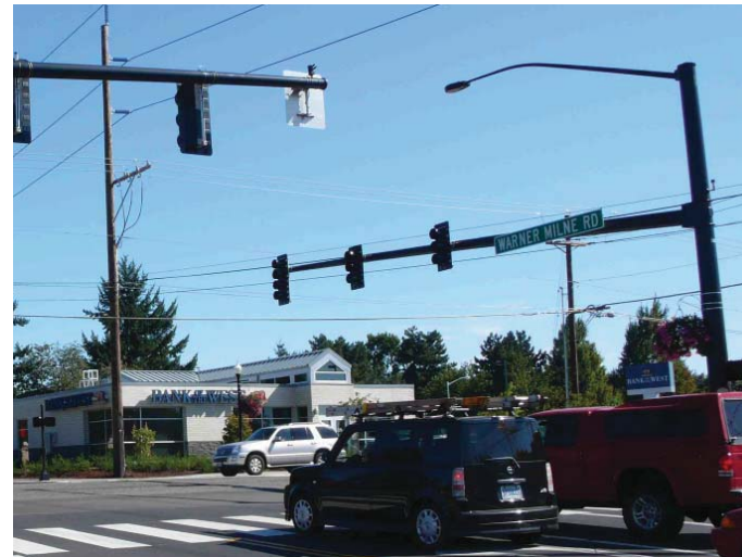
ORNAMENTAL SIGNAL POLES AND MAST ARM EXAMPLE
