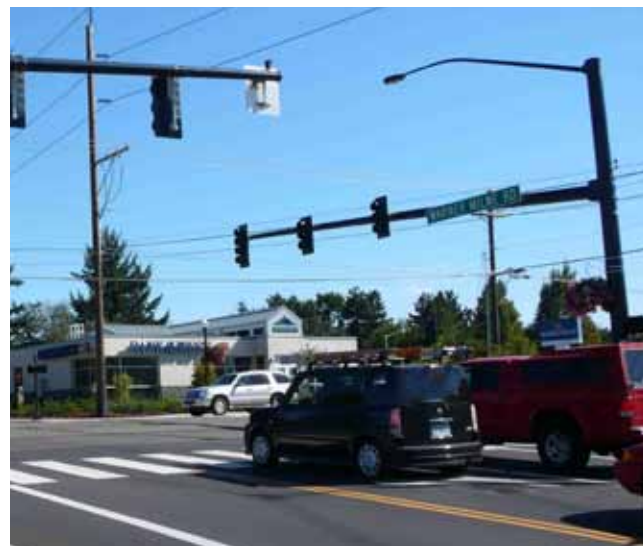
ORNAMENTAL SIGNAL POLES AND MAST ARM EXAMPLE
