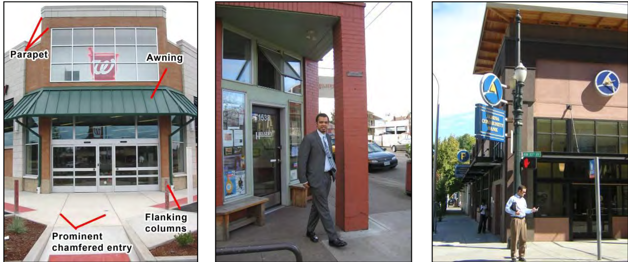
Figure 63 Corner of building elements
