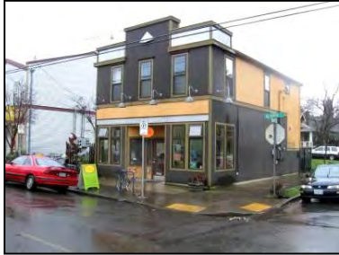
Figure 32 Top of building features a parapet
