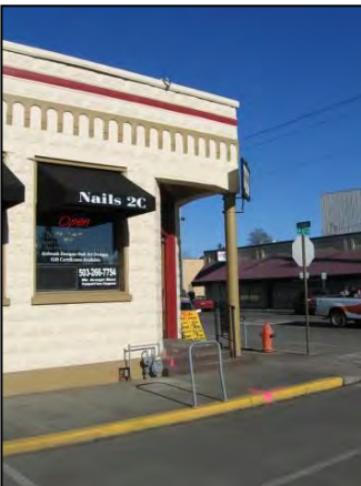
Figure 31 Cornice details near the top of building
