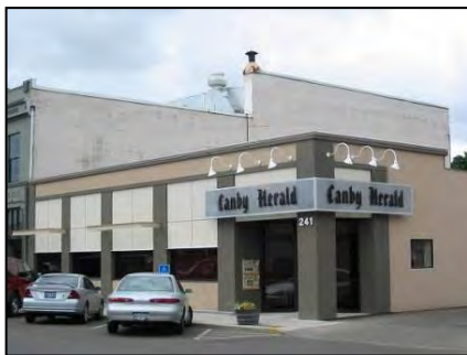
Figure 24 The Canby Herald Building in the commercial core incorporates many good design elements including a recessed entry, sign frieze, engaged columns and decorative lighting
