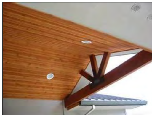
Figure 42 Recessed entry with lighting and accent material
