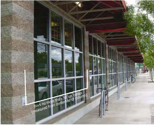
Figure 29 Repeating bays with a continuous awning
