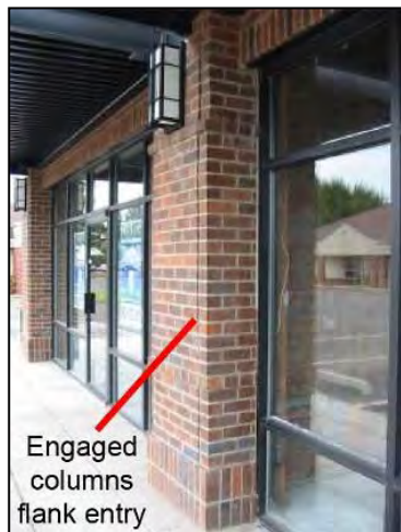
Figure 43 Entry flanked by engaged columns and lighting
