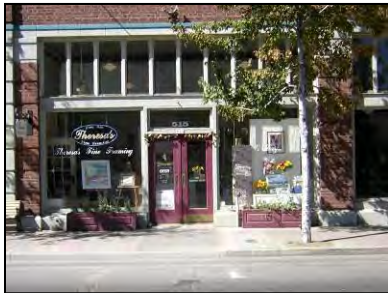
Figure 33 Building entry features a transom window above the door
