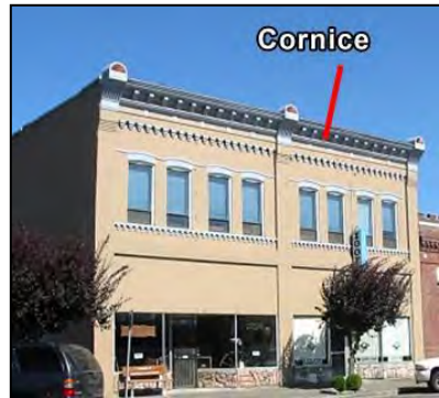
Figure 58 Cornice used on flat roof
