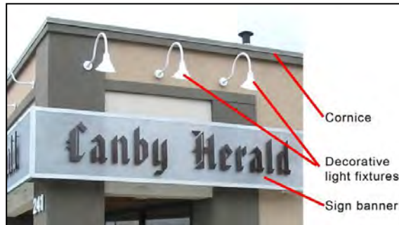
Figure 55 Middle and top of ground floor elements
