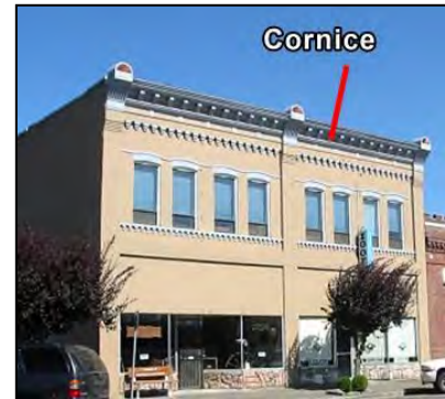
Figure 58 Cornice used on flat roof
