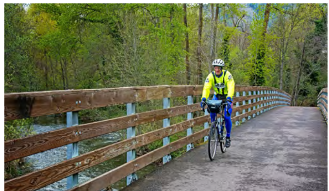
A bicycle and pedestrian bridge can link the area’s neighborhoods across Willow Creek
