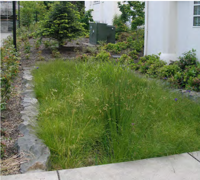
Typical LIDA facilities: Residential rain garden
