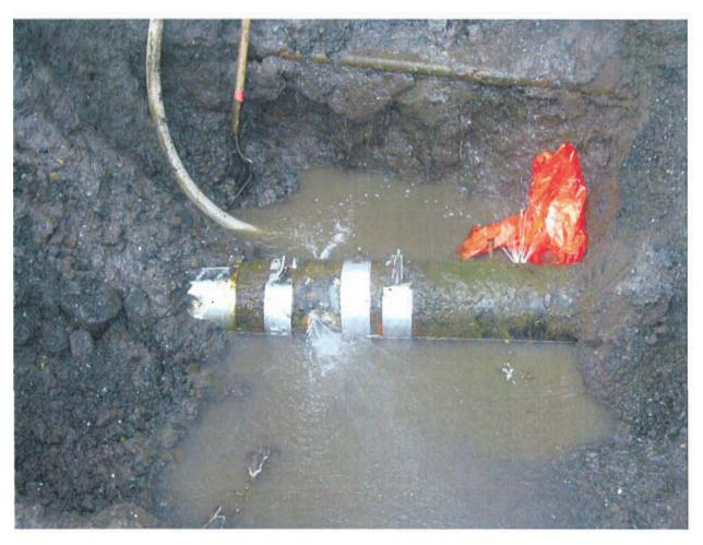
Note the number of repair bands already existing prior to the work to fix the three new leaks.
