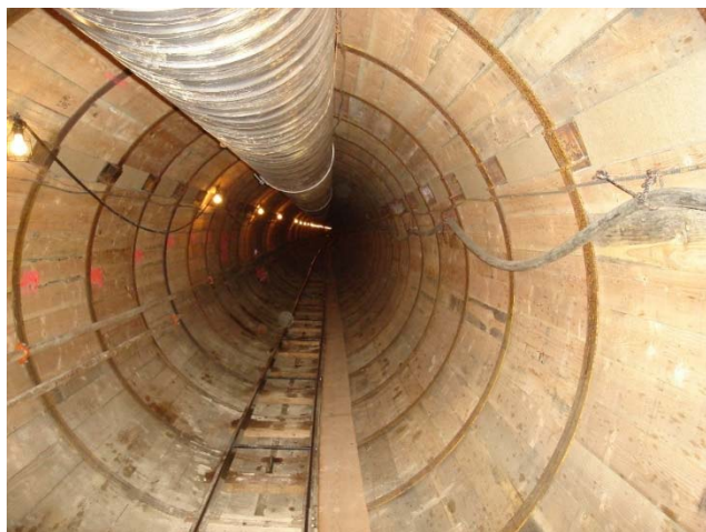
EXHIBIT D Example of Ribs-and-Lagging Support Source: CH2M
