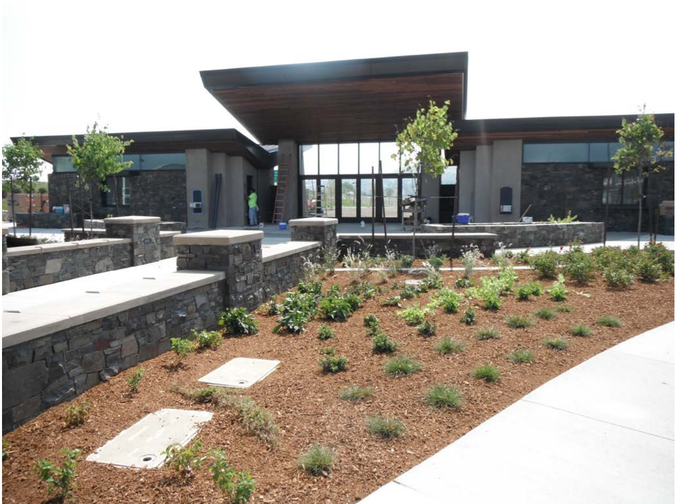
New concession and restroom building in the new Lewis & Clark Festival Area constructed in FY11/12.
