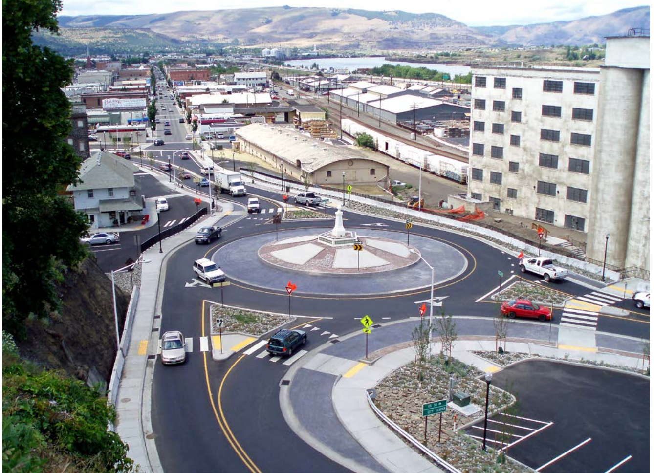
Round-a-bout constructed in FY09/10
