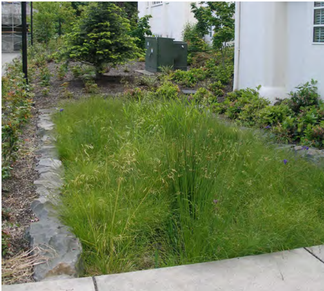
Typical LIDA facilities: Residential rain garden
