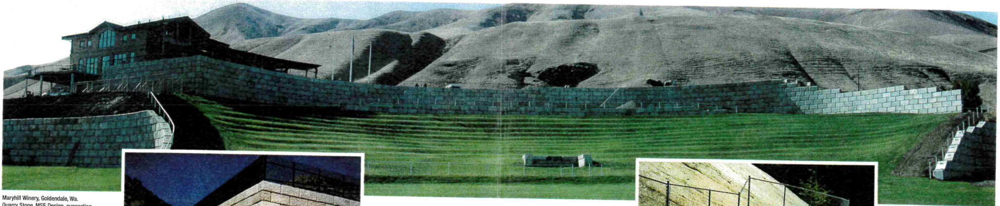
Maryhill Winery, Goldendale, Wa. Quarry Stone, MSE Design, supporting the outdoor visitor's wine tasting area and surrounding amphitheater.
