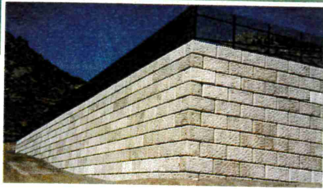
Nevada D.O.T. Maintenance Yard Virginia City, NV. Quarry Stone, MSE wall built to expand storage area.
