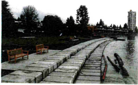
Vancouver Harbor, Vancouver BC. Block steps provide the perfect transition between the pedestrian walkway and the water front.
