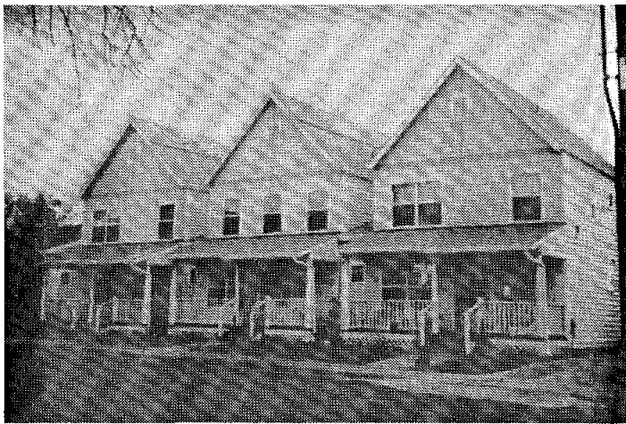
Attached dwellings which appear similar to surrounding single-family dwellings, Portland, Oregon
