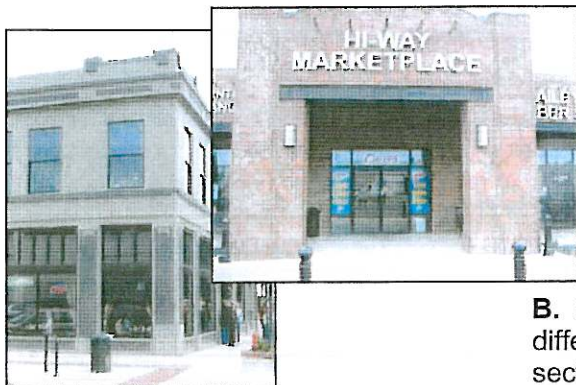
Figure 8 These buildings in the commercial core illustrate desired design features in that area
