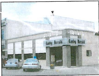
Figure 8 The Canby Herald Building in the commercial core incorporates many good design elements including a recessed entry, sign frieze, engaged columns and decorative lighting
