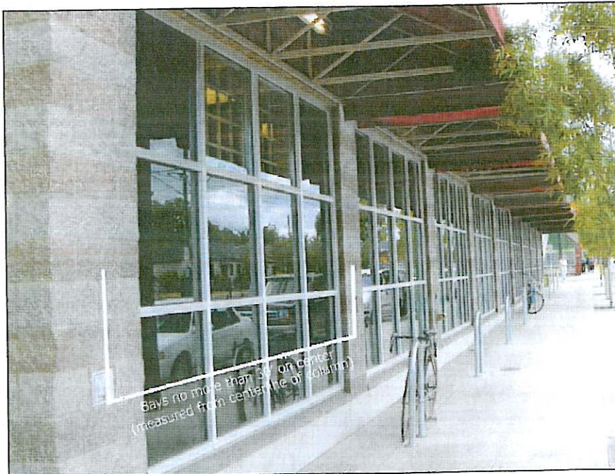
Figure 13 Repeating bays with a continuous awning
