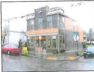
Figure 17 Top of building features a parapet
