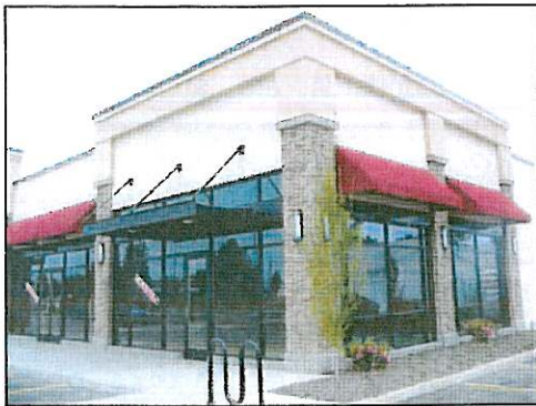
Figure 6 Use of materials such as stone and stucco add to a feeling of permanence
