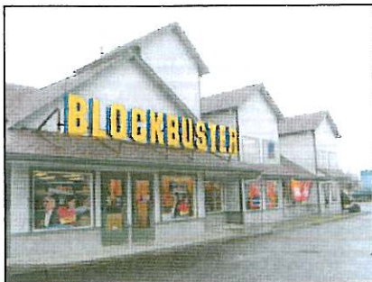
Figure 16 Multiple gable roof elements
