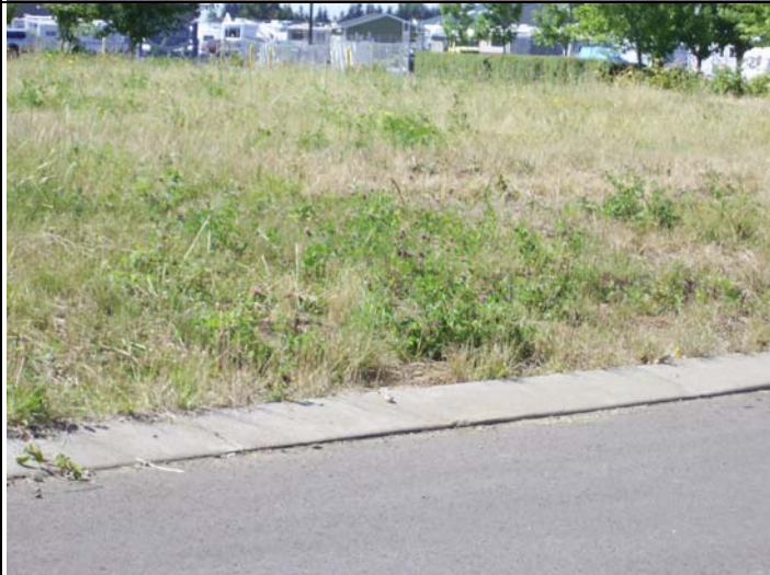
③ Photo shows the existing rolled curb that has already been constructed along the lot line abutting the shared driveway.
