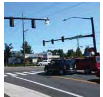
Ornamental Signal Poles and Mast Arms
