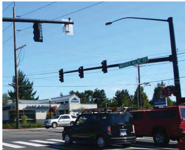
ORNAMENTAL SIGNAL POLES AND MAST ARM EXAMPLE
