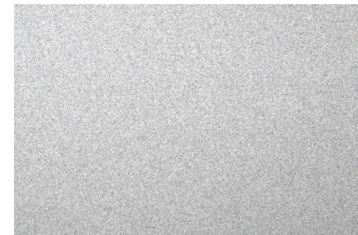
Modified Bitumen Roof with White Cap Sheet
