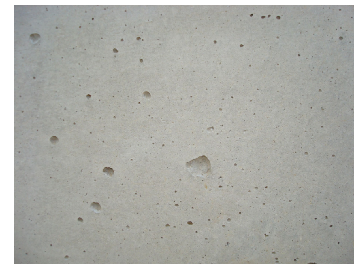
Concrete Base & Bulkheads
