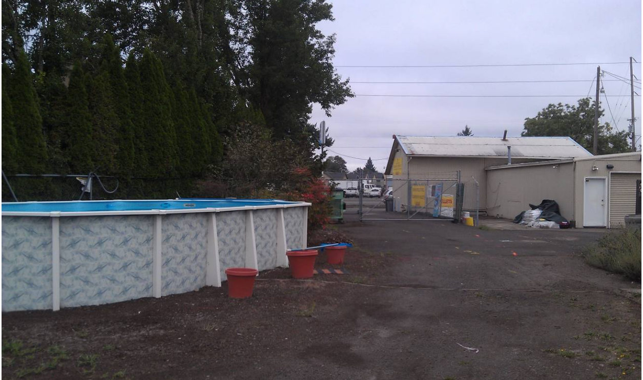
Swimming pool and unpaved southern area at Classic Pool and Spa at 701 SW 1st Avenue. Tan building is Classic Pool and Spa retail store. Pool chemicals can be seen on palettes adjacent to store. Photograph taken looking north.
