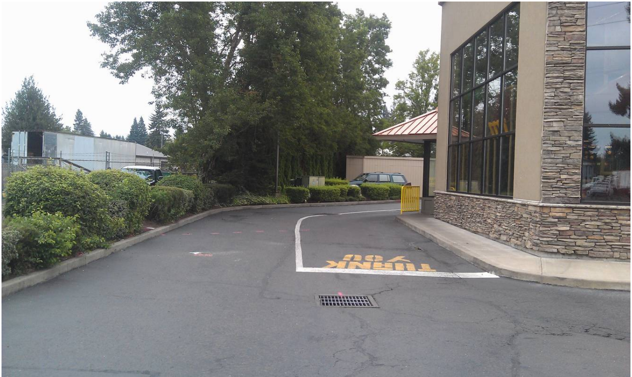
Drive-thru lane at McDonald's restaurant at 709 SW 1st Avenue. Storage trailer at Classic Pool & Spa is visible in left background of photo. Photograph taken looking south.
