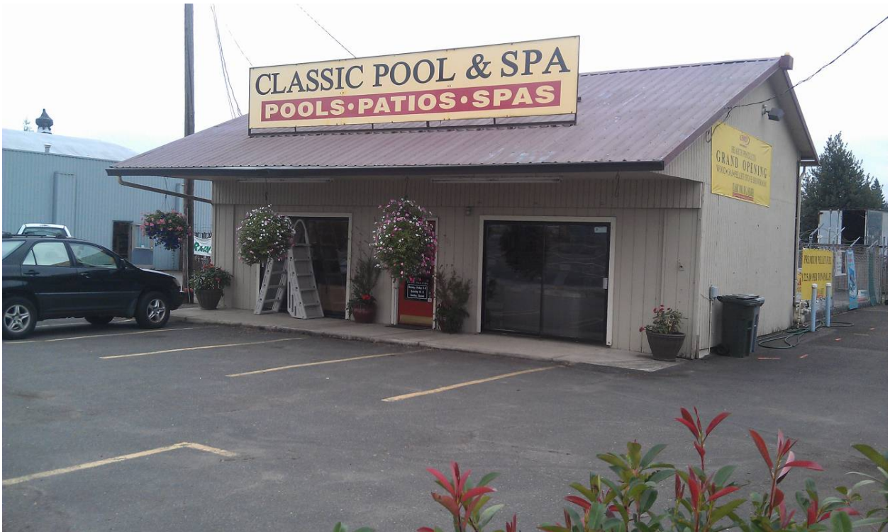
North and west side of Classic Pool and Spa building at 701 SW 1st Avenue. Photograph taken looking southeast.
