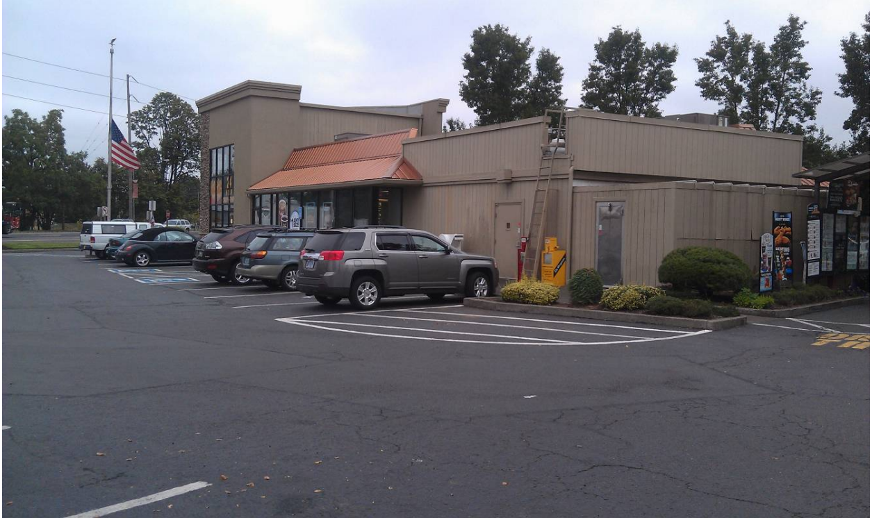
Southwest corner of McDonald's restaurant at 709 SW 1st Avenue. Photograph taken from parking lot looking northeast.
