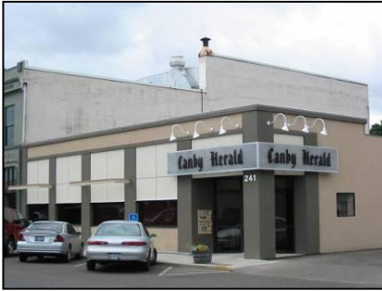
Figure 24 The Canby Herald Building in the commercial core incorporates many good design elements including a recessed entry, sign frieze, engaged columns and decorative lighting
