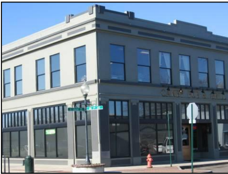
Figure 19 Design details such as a recessed entry, columns and decorative transom windows help articulate the ground floor and distinguish it from the upper floors
