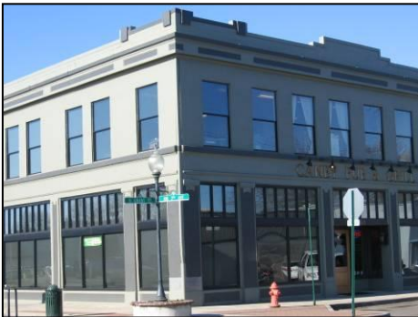
Figure 19 Design details such as a recessed entry, columns and decorative transom windows help articulate the ground floor and distinguish it from the upper floors
