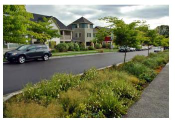
Bioswales in a residential development treat stormwater runoff from the street and sidewalk.
