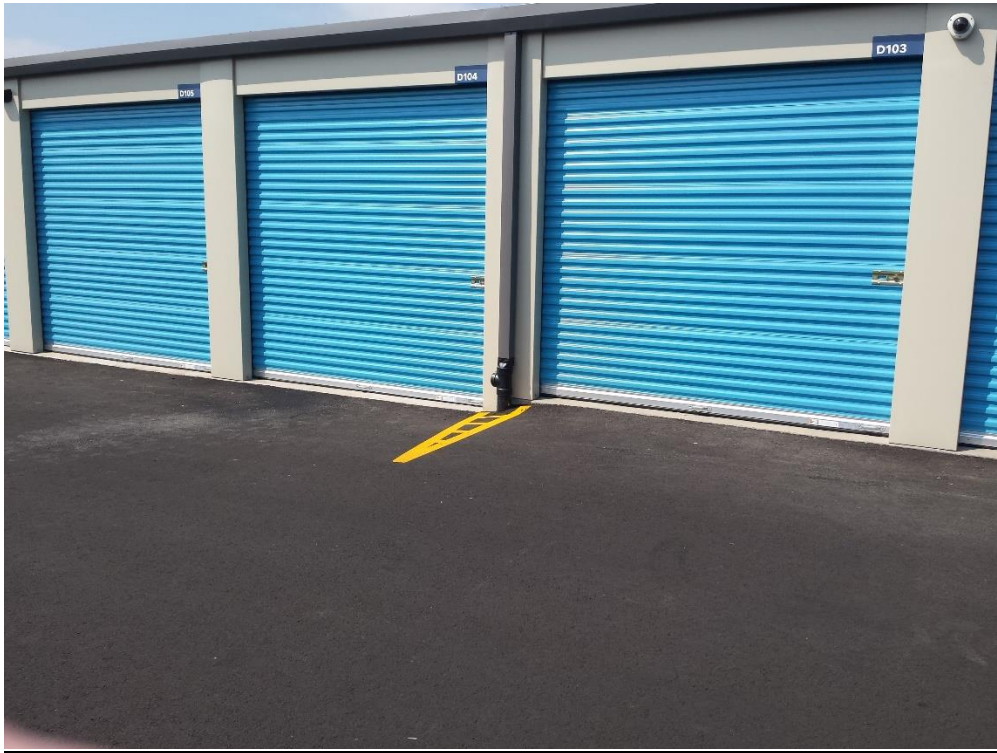
Photo Example of metal doors, metal door jamb "pilasters" and metal headers.
