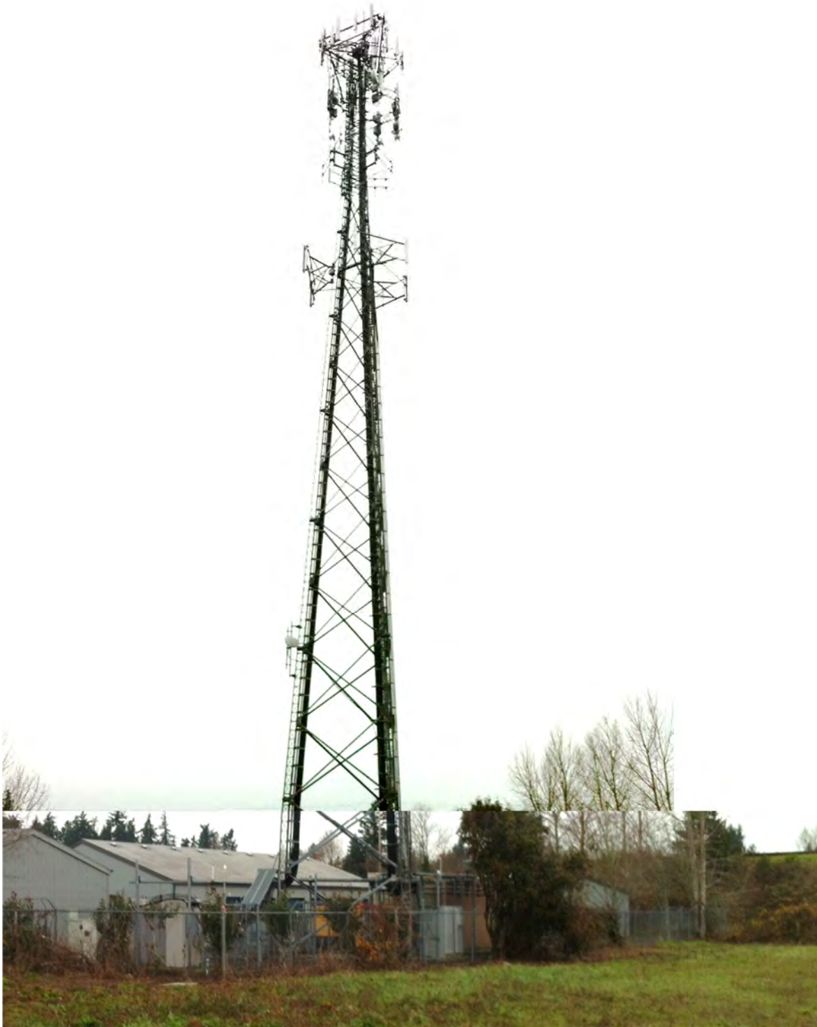
Cell tower and Northwest Self Storage located to the northwest
