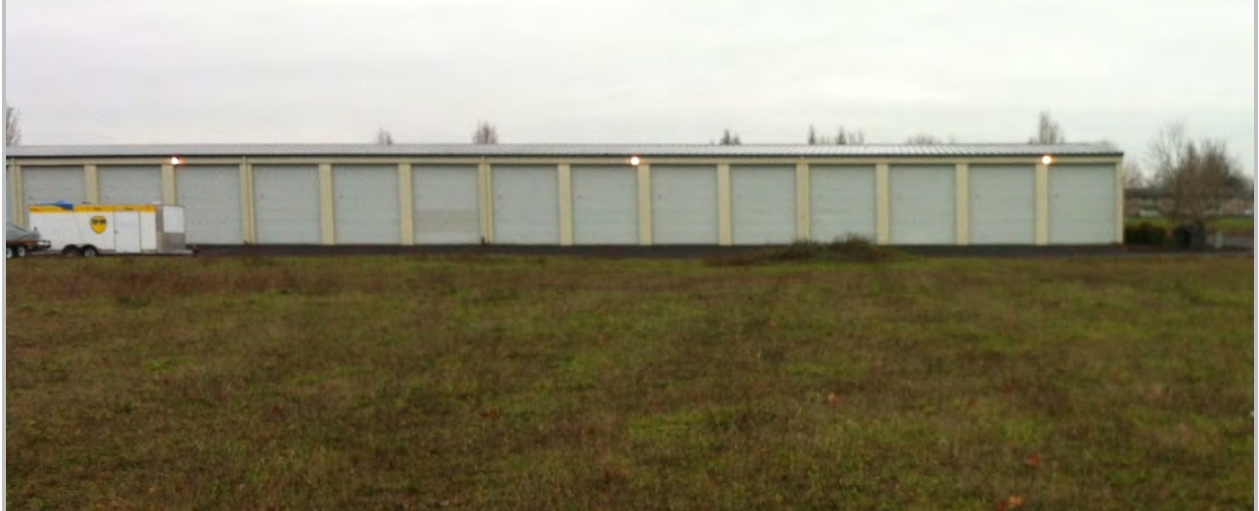
Existing Western Storage building located to the south
