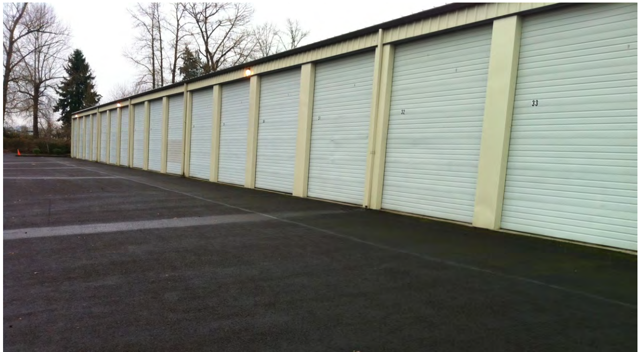
Existing Western Storage building located to the south
