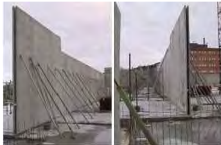
TILT-UP WALL CONSTRUCTION
