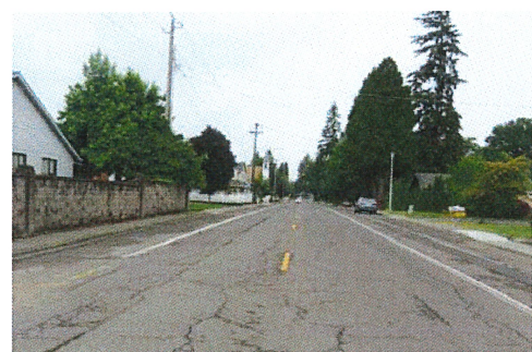
Figure 1: Existing Soundwall along S Township Rd
