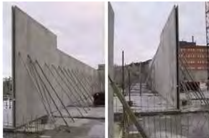
TILT-UP WALL CONSTRUCTION
