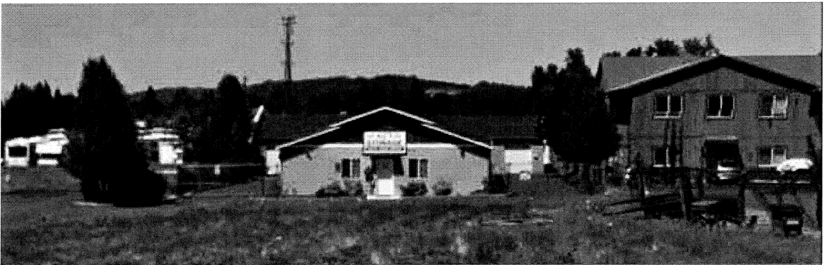
Existing ACT Storage building located to the North. This building is constructed with horizontal composite siding and composite shingle roofing. The southern elevation has an entry door and two windows, the eastern and western elevations are mostly garage doors and horizontal siding.
