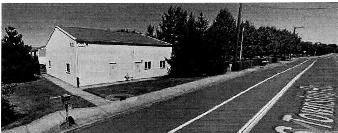
Existing Clear Creek Forest Products building located to the East. Building constructed with vertical metal siding exterior walls and roofing. The southern elevation has a two exterior doors and two small windows. West and Eastern elevations are mostly siding with two windows.
