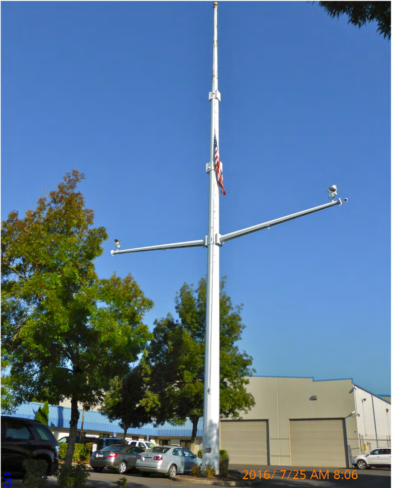
CANBY ID 14, Existing WCF at 1190 NW 3rd Ave, facing 3rd Ave
