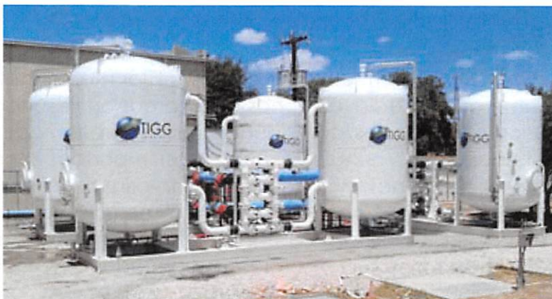
Figure 12 – GAC Pressure Vessels (courtesy of TIGG)
