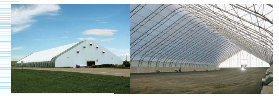
Titan Coverall covers do not contain any metallic components, therefore, it will not rust from exposure to water and air. The steel framework of building is constructed with triple coated corrosion barrier, lasting 270% longer than standard galvanized steel.
