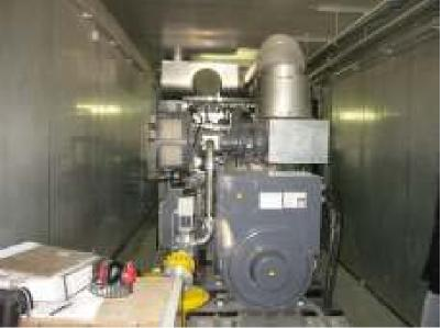
The CHP unit is shipped to the sight in a soundinsulated container. The unit processes the methane into electricity, which is then sent to the grid. It also captures heat which is reused on site.
