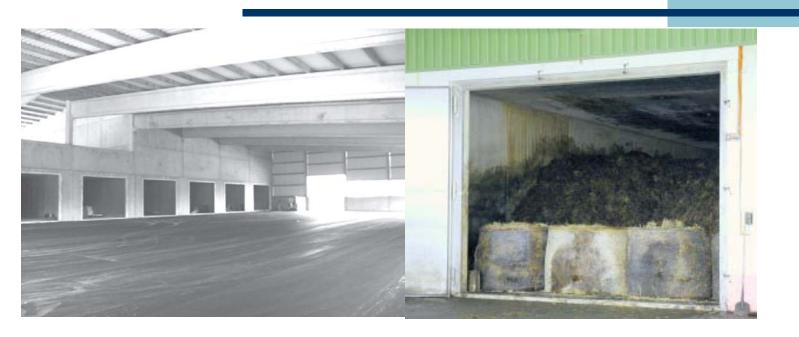
Organic input remains stationary throughout process, eliminating moving parts and resulting in low system maintenance and repair costs. Cells are air-tight and gas-tight. Methane sent to CHP unit.
