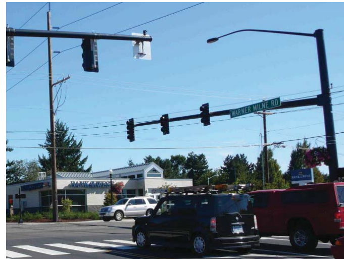
ORNAMENTAL SIGNAL POLES AND MAST ARM EXAMPLE
