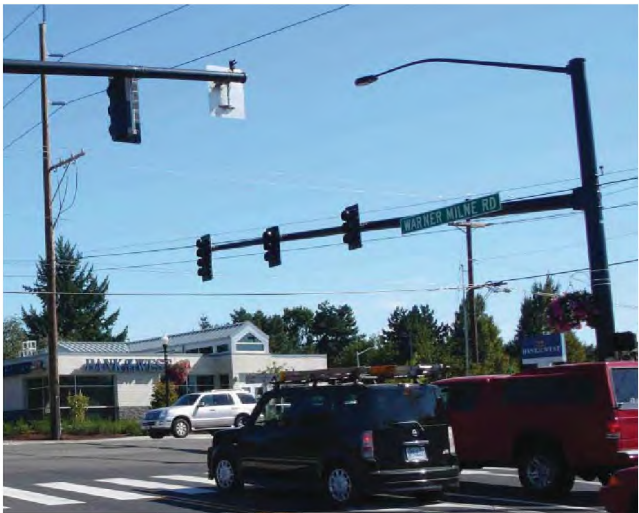
ORNAMENTAL SIGNAL POLES AND MAST ARM EXAMPLE
